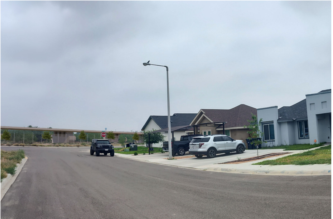
Figure M-5. KOP 1 After Construction of the Northern Rail Alternative, Without Train Traffic (Approximately 550 Feet from Viewpoint)
